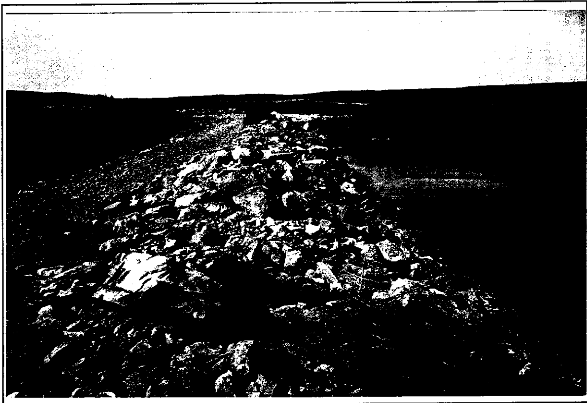
Upstream face showing riprap.
